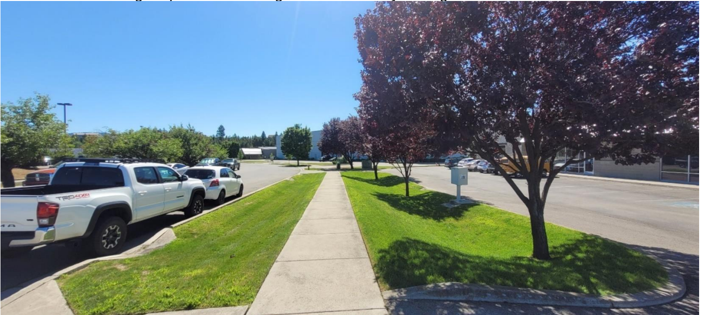
Frontage improvements along N. Schreiber Way looking southeast:
