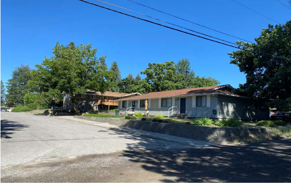
SITE PHOTO - 6: View from western edge of the subject property looking west toward Stiner Ave.
